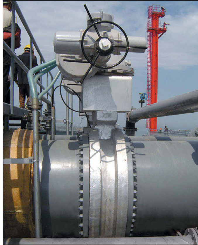
A large Torqseal™ triple-offset valve used for crude oil service in the Dalian Seaport (China).
