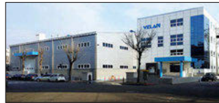
Ansan City, South Korea Velan Ltd., Plant 1
