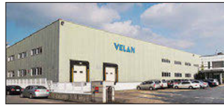
Ansan City, South Korea Velan Ltd., Plant 2
